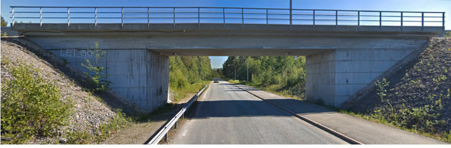
Fig. 10. Hörnefors railway bridge.
